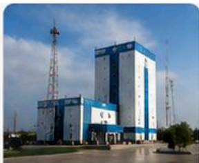
Installation and refueling complex
